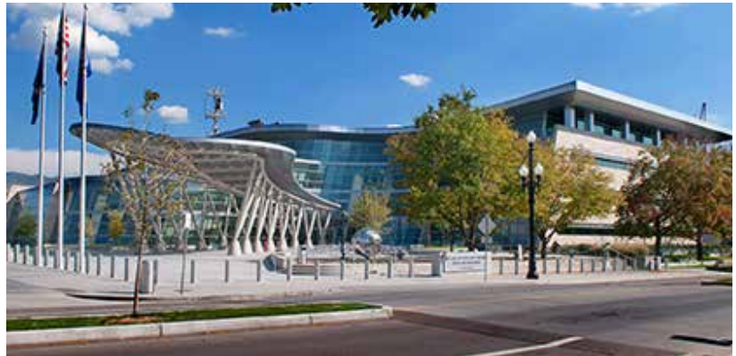
Critical equipment in the Salt Lake City Public Safety Building in Utah, USA is protected by an extensive DIS Isolated Platform System.
