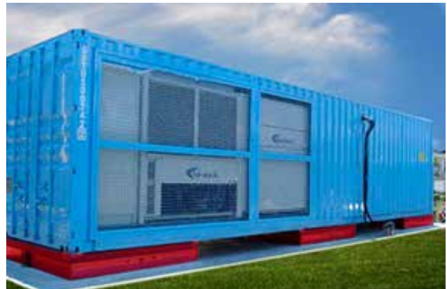
Modular Data Center In Costa Rica. It performed well in a 2012 magnitude 7.6 earthquake.
