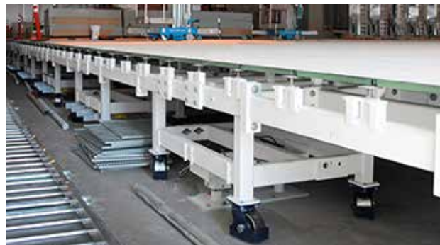
Installation of a 16,000 square foot isolated floor at the UC Berkeley, Computational Research and Theory Facility.
